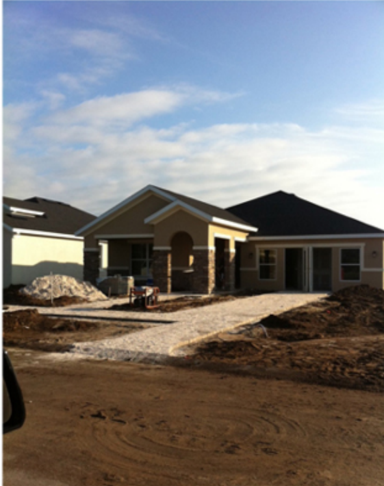
Residential construction by KB Homes in LPGA International
