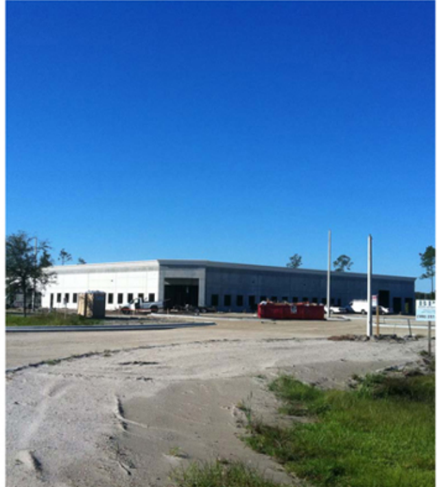
Commercial construction for Ark Technologies in Gateway Center
